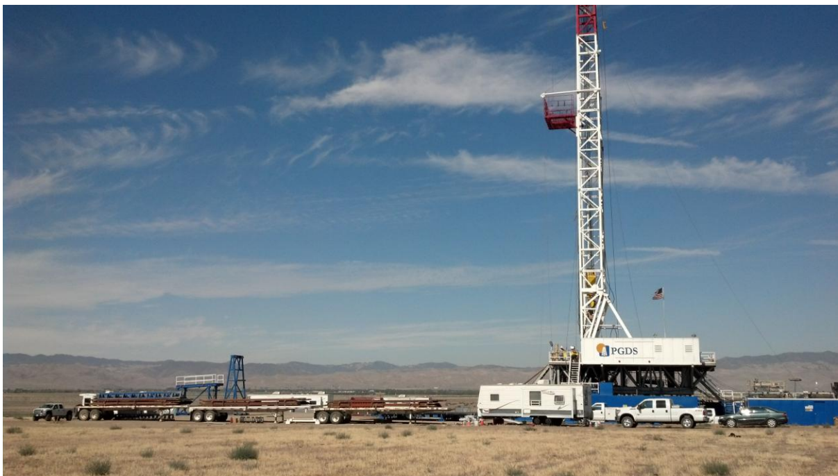
Graham Drilling Rig 5 looking west
