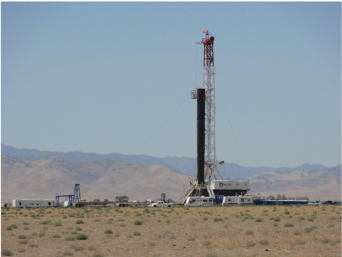
Graham Drilling Rig #5
