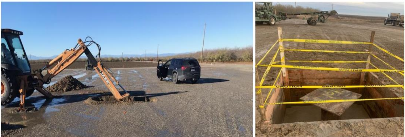
Fig. 1: Borba 1-7 Well Cellar Construction
