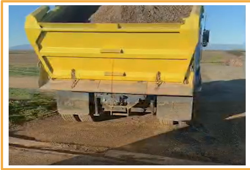
Fig 4: Truck laying road to Borba Drilling Pad Site
