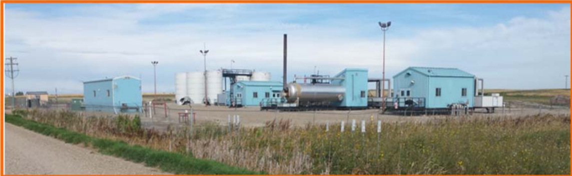
Representative Asset Oilfield Production Facilities (Little Bow Oilfield Battery)
