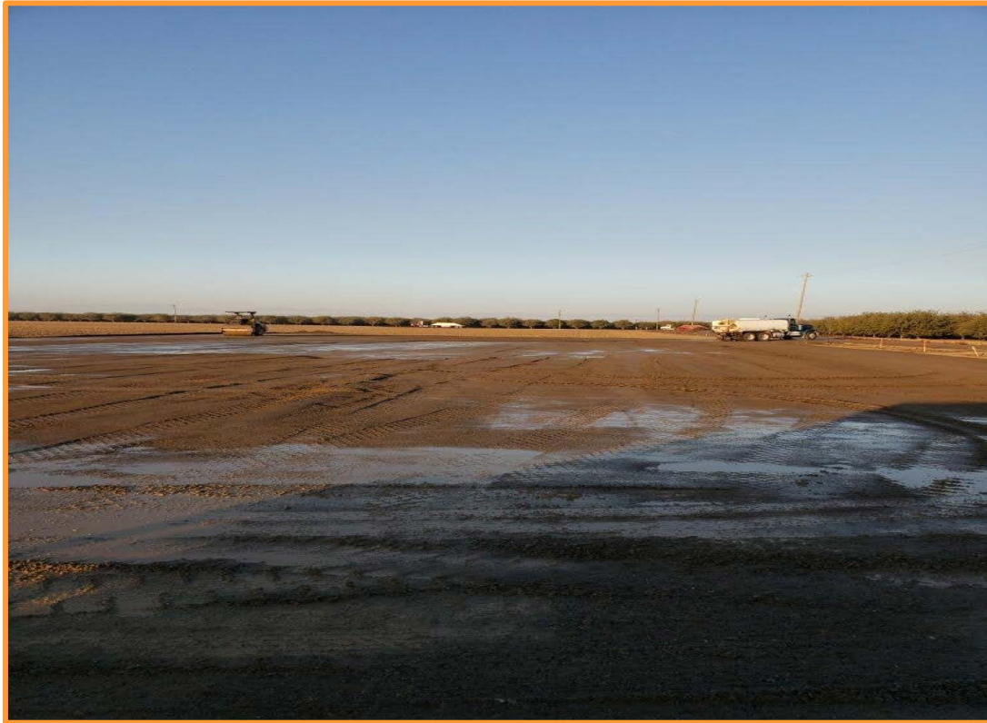
Borba 1-7 Well Pad and Production Platform Ready for Drilling Rig
